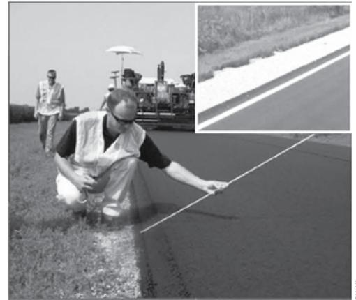
*This shows the Safety Edge during an overlay project and the finished product with the shoulder material in place next to the Edge (inset).*
