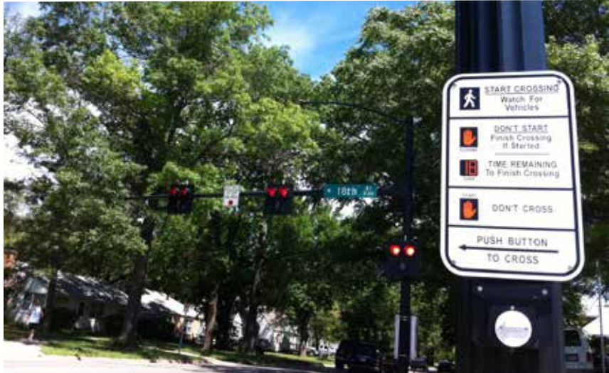
When activated by a pedestrian, this Pedestrian Hybrid Beacon at 18th and Kentucky Streets in Lawrence stops traffic to allow school children to cross the street near Cordley Elementary School.
