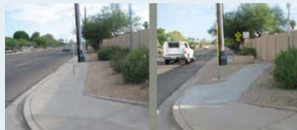
Before and after: Sidewalk obstructed by pole was re-aligned.
