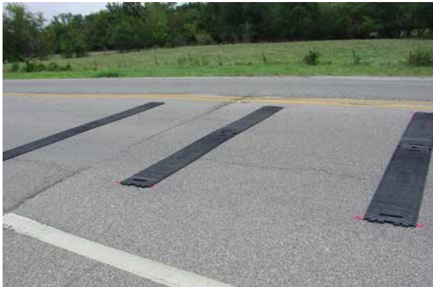
KDOT places the rumble strips in advance of the action warning sign at a work zone. The idea is that drivers will hit the strips and look up to see the sign.
