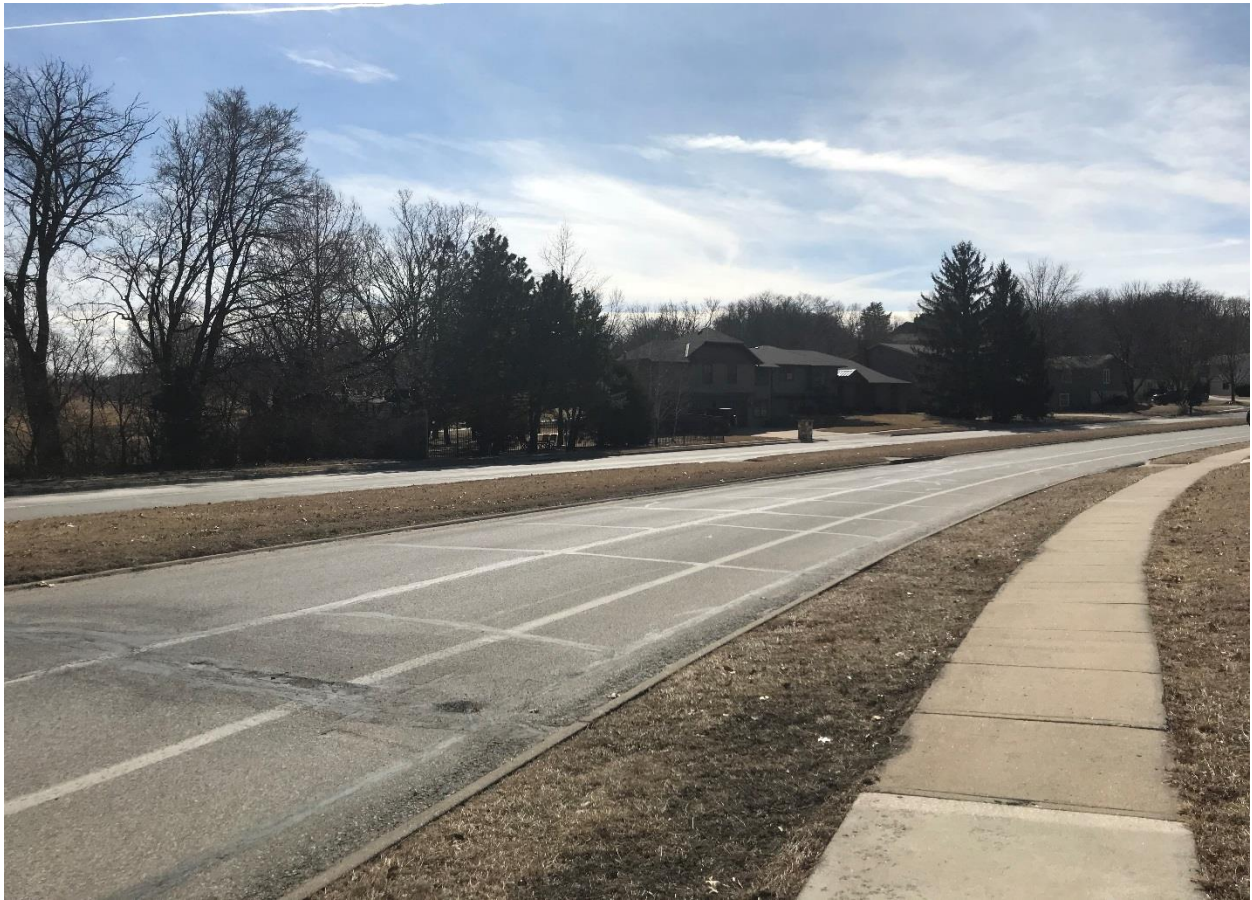
An example of a quick-build project with a drive lane, a buffer, and a bicycle lane. Lawrence Avenue at Princeton Avenue in Lawrence, KS.
