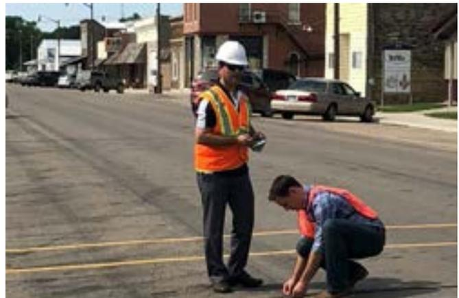
Figure 1. Kansas LTAP Team Installing Pneumatic Road Tube Counter in Republic County, Kansas.
