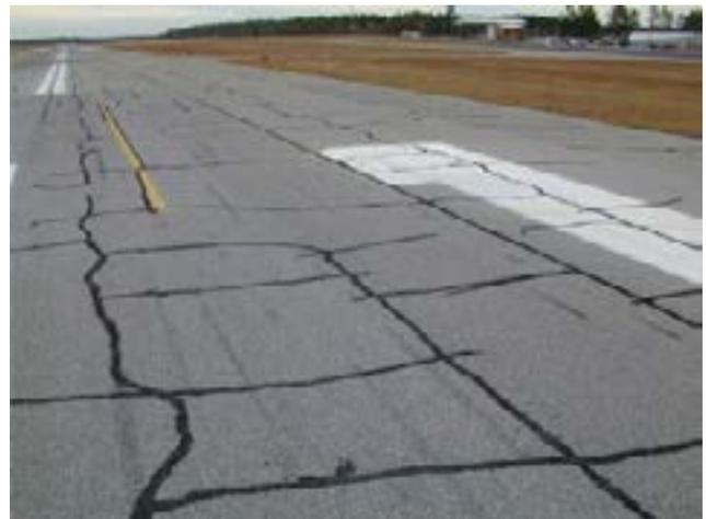
Block cracking plagues county roads. Above is an example of a low distress road from Iowa's Department of Transportation.
