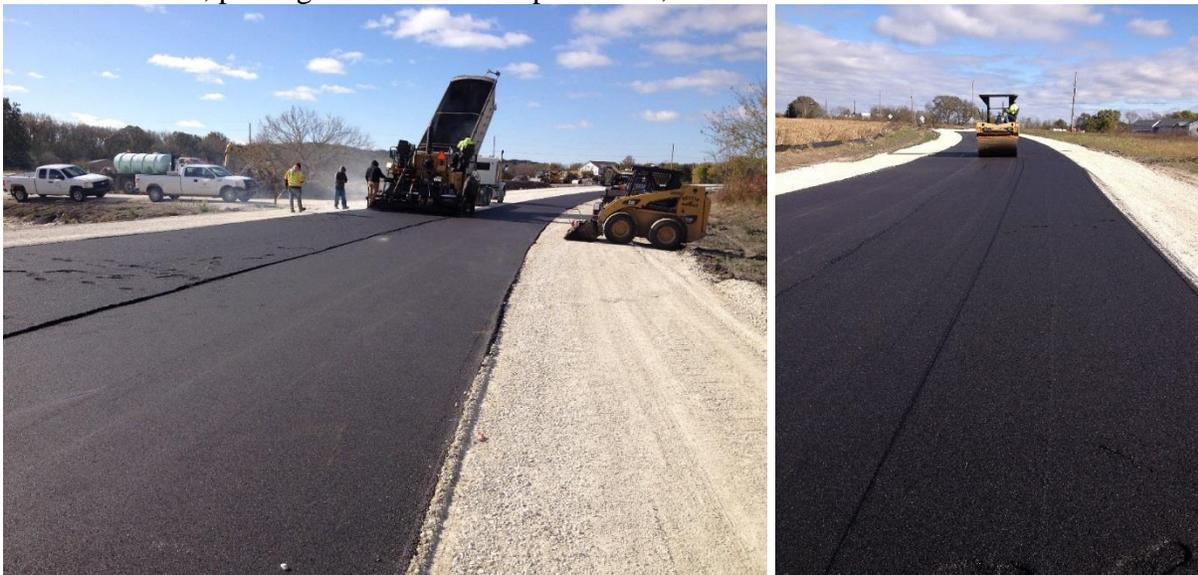
N1000 and E1000, placing and compacting the second lift of asphalt
