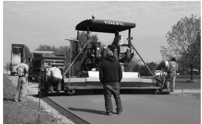
Mystic Lakes project, Maize, KS, Courtesy of Andale Paving, Inc.
