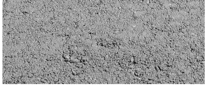
Close-up, the texture of RCC is similar to asphalt.
