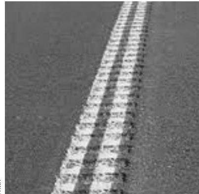
*Painted center line rumble strips are especially helpful in conditions of low visibility. Besides creating noise and vibration, the strips are more visible than typical painted lines because of the raised surface.*
