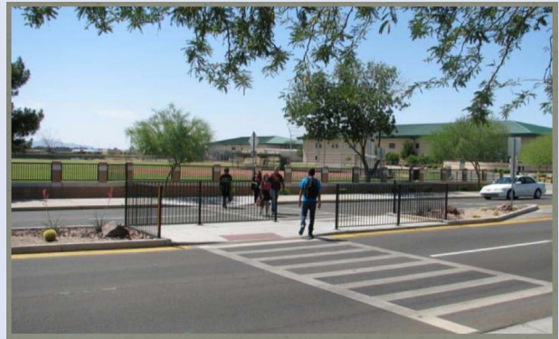
A midblock crosswalk was designed to accommodate students crossing an arterial to get to food establishments. Students were not using the pedestrian crossing 600 ft. away.
