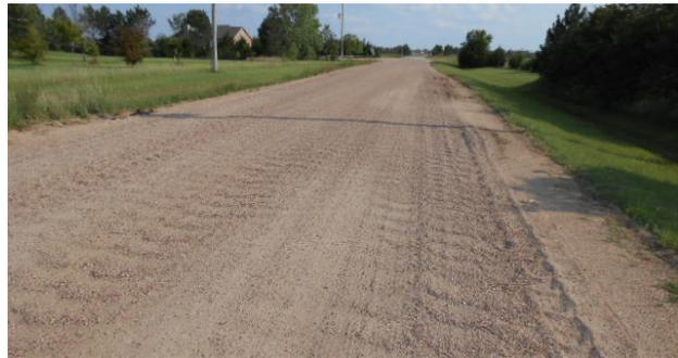
Fig 9. Washboards are common in dry weather.
