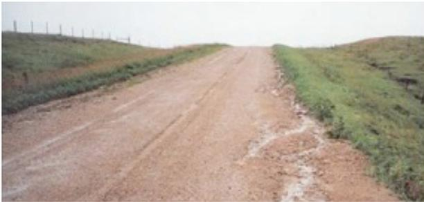
Fig 4. High shoulder causes erosion along edge of road.
