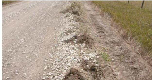
Fig 6. Improper mixing of dirt with windrow when repairing a high shoulder.
