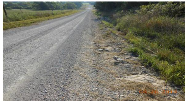
Fig 7. Inadequate ditch evidenced by washing along shoulder.
