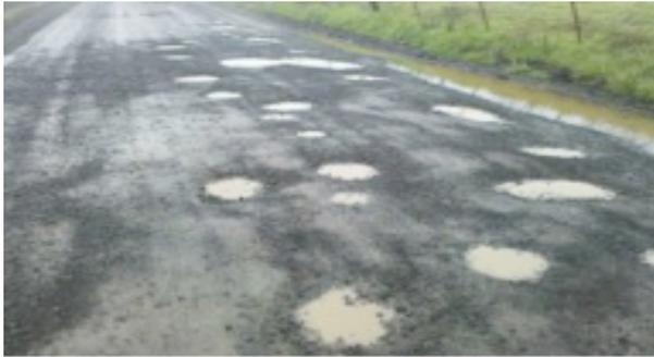
Fig 8. Potholes caused by inadequate cross slope at a low spot.
