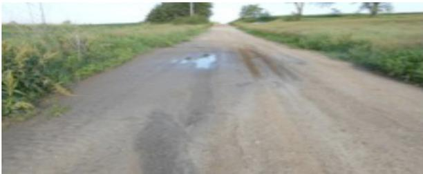
Fig 5. High shoulder causes mud hole at low spot.
