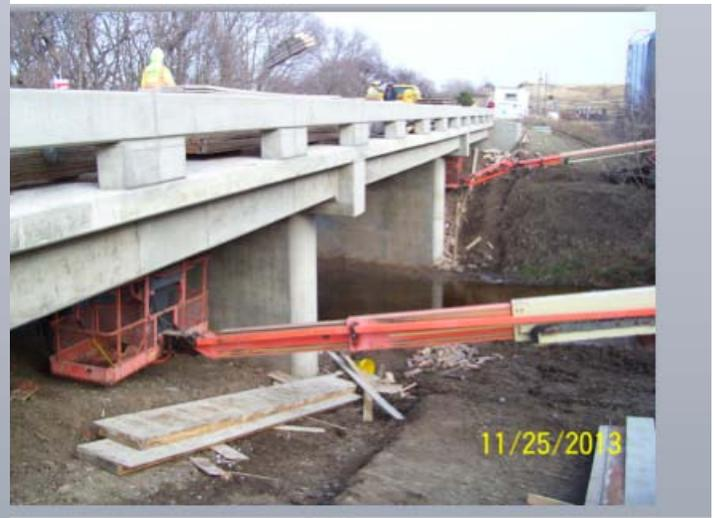
**At left,** placement of formwork and supplemental reinforcing around existing steel beams in preparation for concrete placement.
