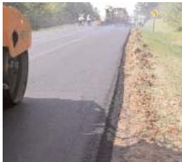
Asphalt pavement contractors can use a special edging device on resurfacing equipment to install the "Safety Edge" while resurfacing. The roadway shown above was placed by the Georgia DOT using the "Safety Edge."
