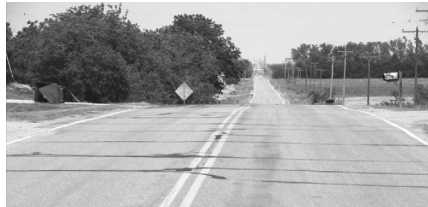
Light repair for hot mix roads: Latex modified slurry seal, before (left) and after (right).
