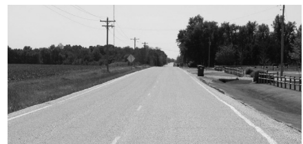
Repair for cold mix roads: Skim coat and chip seal, before and after.
