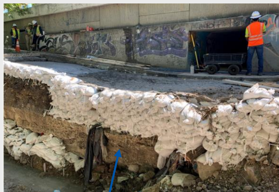
Concrete Encased Water Line
