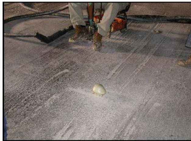
Figure 5.18 URETEK Slab Jacking Process
