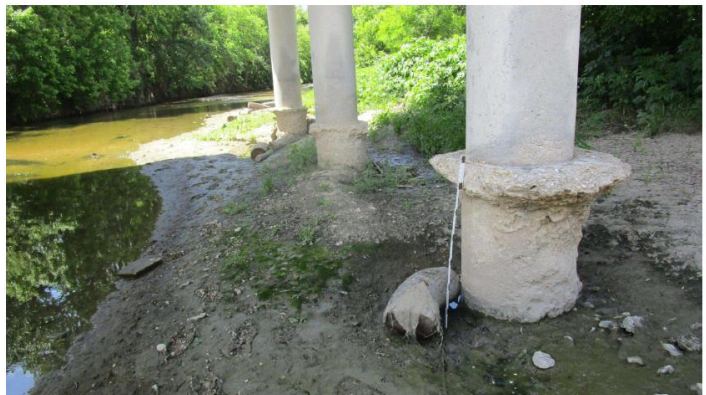
PHOTO 10 Description 10_Bent 5 drilled shafts are exposed 3 ft high (Looking South)
